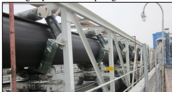
Fig 2: Pipe conveyor at NTECL
