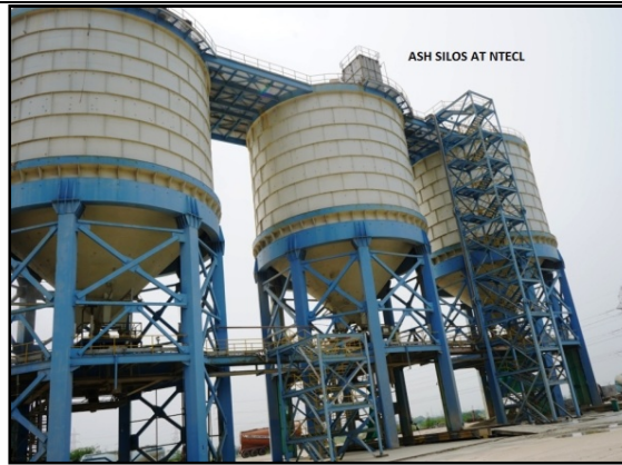
Fig 5: 3 No of Dry ash silos at NTECL
